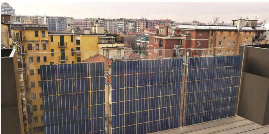
The BIPV products EnergyGlass™ replaces building elements (roofs, facades, balustrades, canopies, etc.) performing a multifunction role: they generate power and are architectural elements of the building envelop.
